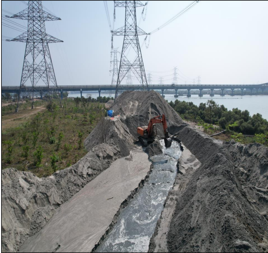
Poclains used in making drying pits
