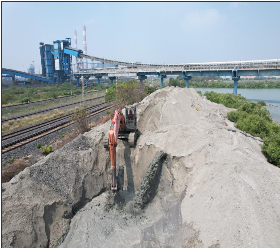
Poclains used in making drying pits
